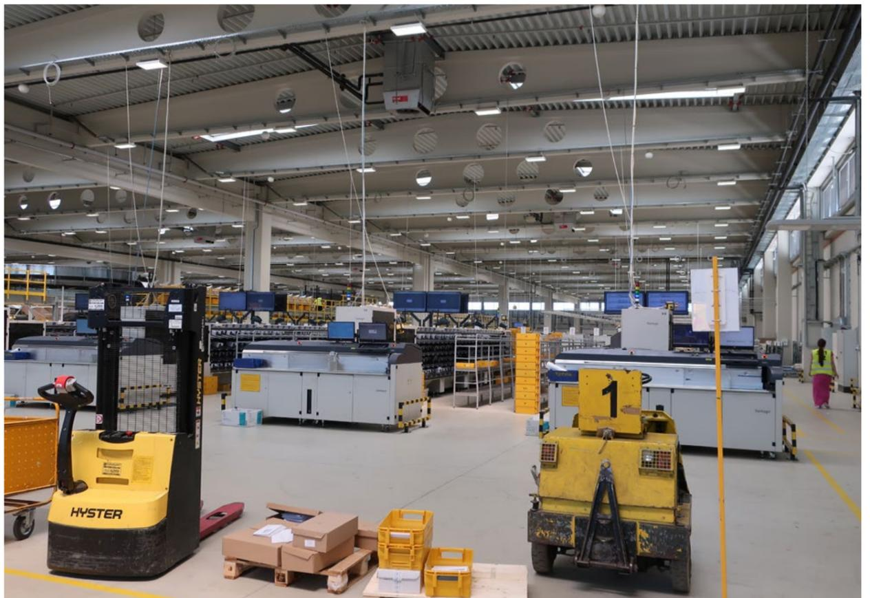
The Croatian Post's 32000 m<sup>2</sup> logistics centre sends parcels all over the country and is a workplace for around 1500 employees. The TopTronic® C control platform manages 14 decentralised RoofVent® and TopVent® supply and extract air handling units to heat the hall and supply it with fresh air.
